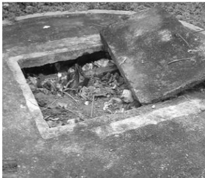
Fig. 2, Open septic tank used as waste disposal in Wonosari (Oertel)
