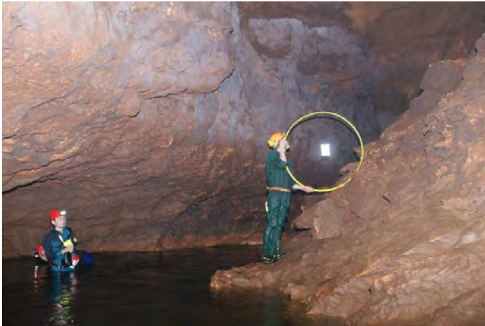
Rock slope with the visualized pipeline in downstream view in section 2
