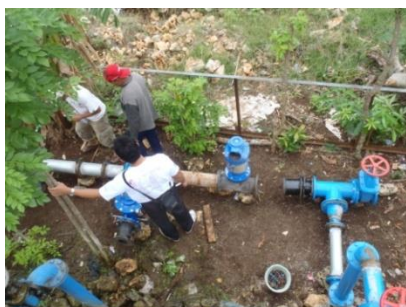
(e) Implementation: installation of control devices
